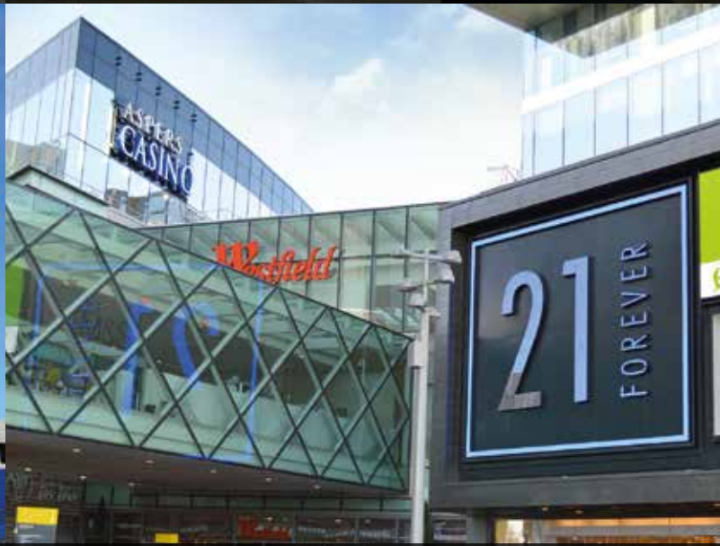
INSTALLATION: WESTFIELD SHOPPING CENTRE, LONDON
